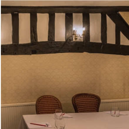
Timber framed walls at The Three Swans.
